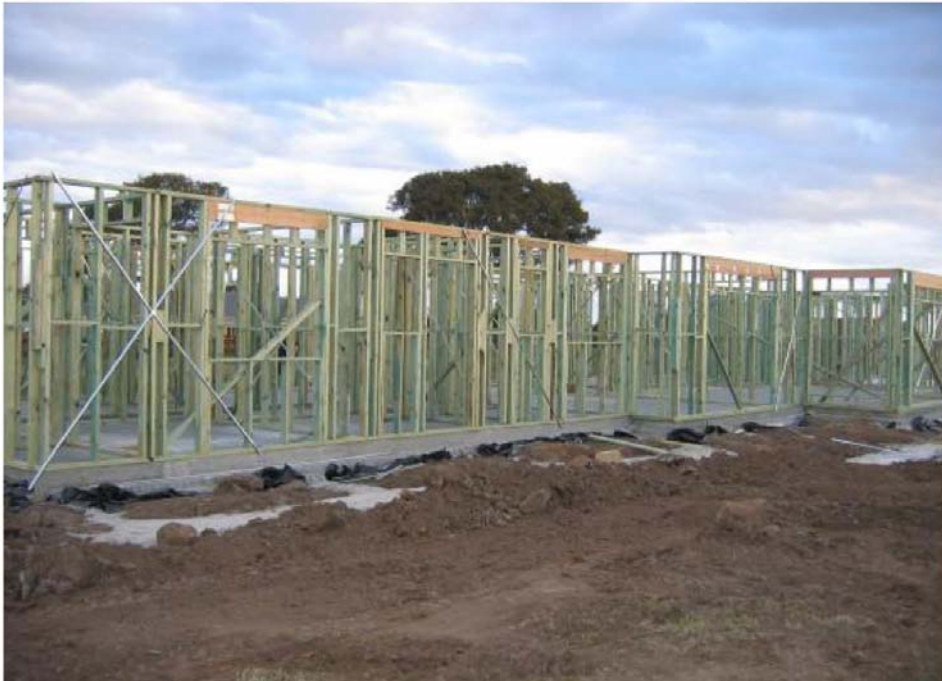
Blue Pine H2F protected roof trusses and wall frames under construction.
